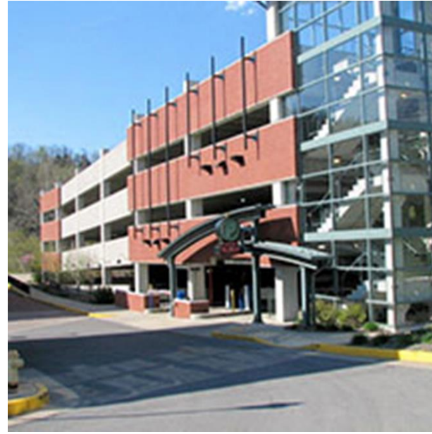
University Avenue / Chestnut Parking Facility (accessible from University Avenue and Chestnut Street)
